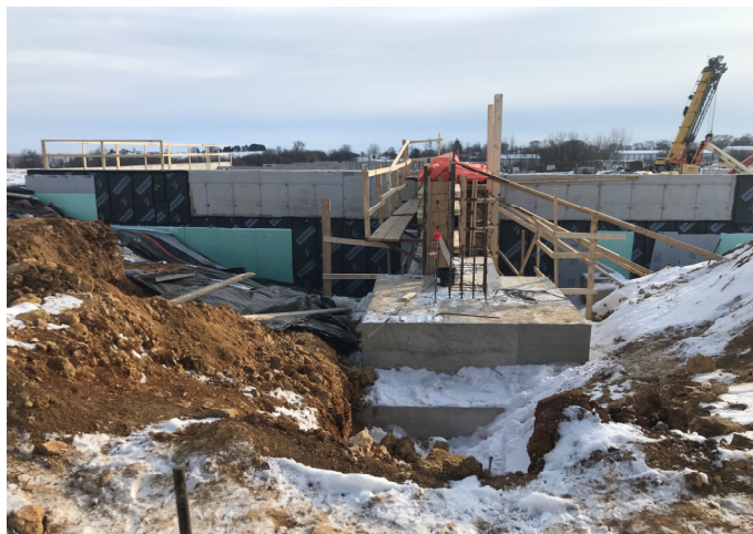
Forming & Pouring Gymnasium Buttress Wall
