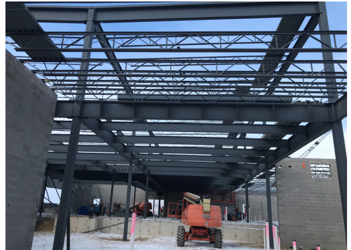
Steel Beams, Joist, Decking & Detailing in the Administration Area
