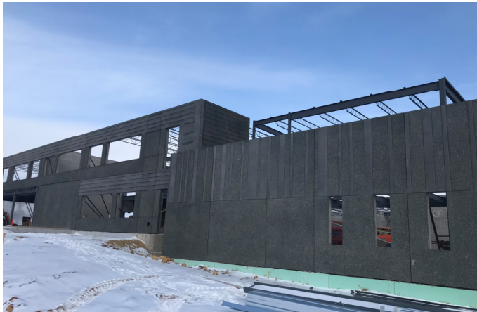
Precast Wall Paneling, Administration & CTE West Elevation
