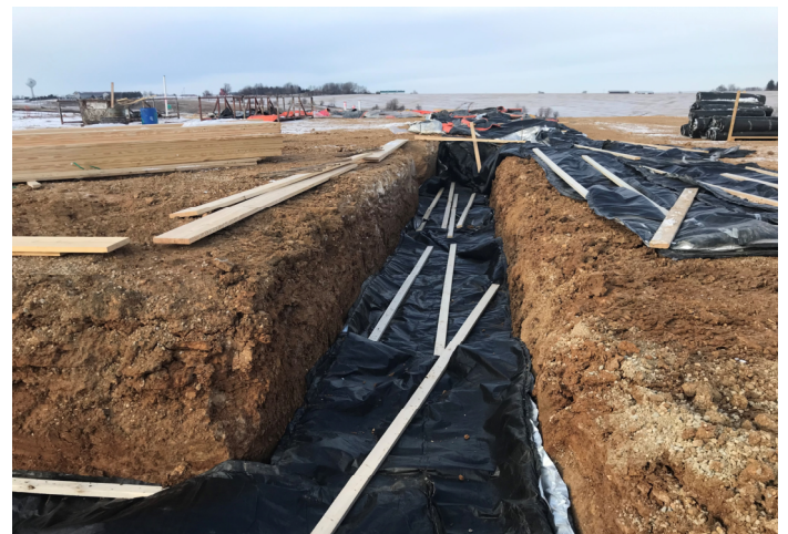
Thawing & Digging Foundation Footings, Auditorium Area
